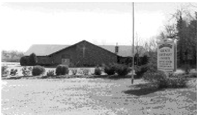
Grace Covenant Church Building Middletown CT. U.S.A.
